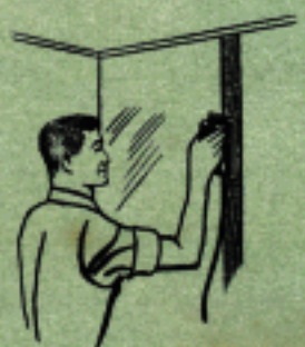
IDEAL FOR SANDING DRY WALL CONSTRUCTION
